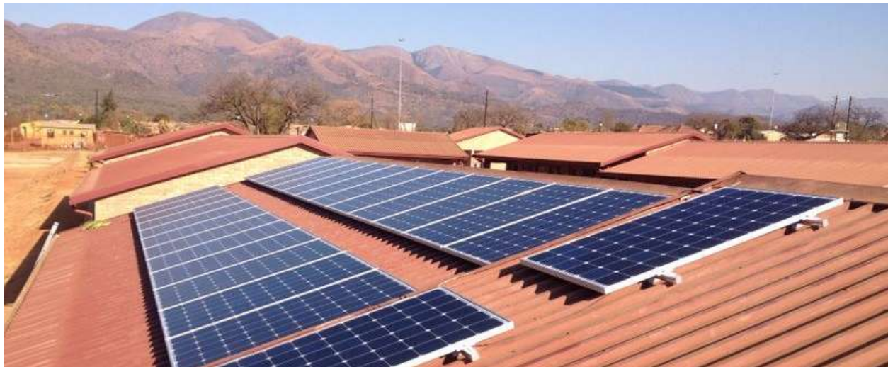
SGP South Africa- 7kw Solar PV Panel installed at the Fairview Primary School in Barberton, Mpumalanga Province, SA
